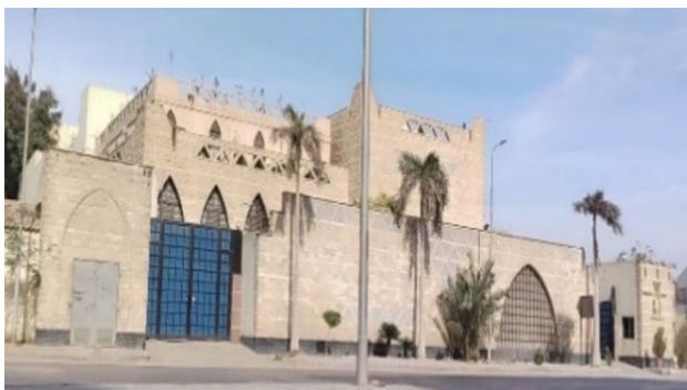
Fig. 25 Waste Management Unit (Source: Authors)
